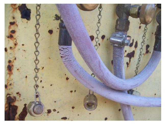
Answer: Hose should be taken out of service due to dry rot & cracking. Also, wrong type of repair clamp (not a high pressure clamp).
