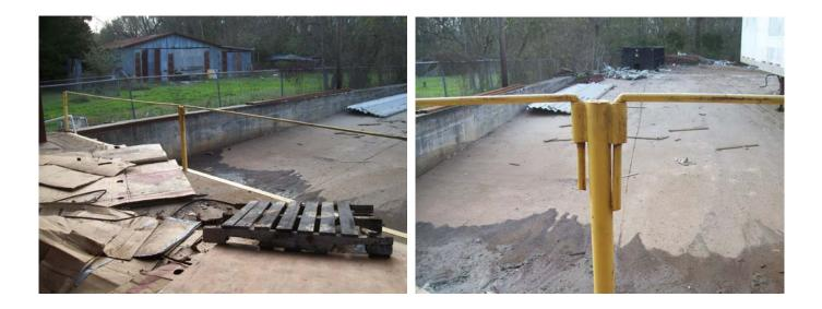
Raised loading docks should be guarded in some way to offer a warning to those near in order to prevent falls. Gates and chains are options. Here's an alternative that comes to us from our friends at Acadia Scrap. Use solid steel rod or rebar inserted into cut pieces of pipe. This set up offers a substantial and inexpensive way to protect people near docks.
